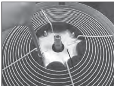
(14) IMPORTANT! Fit new motor mounting nuts & tighten (5Nm S Series or 8Nm FX Series).
