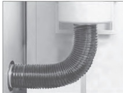
(2) Check any ducting for damage or blockage.
